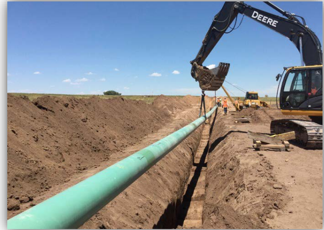
DJ Basin - Empire Pipeline for SRC Energy
